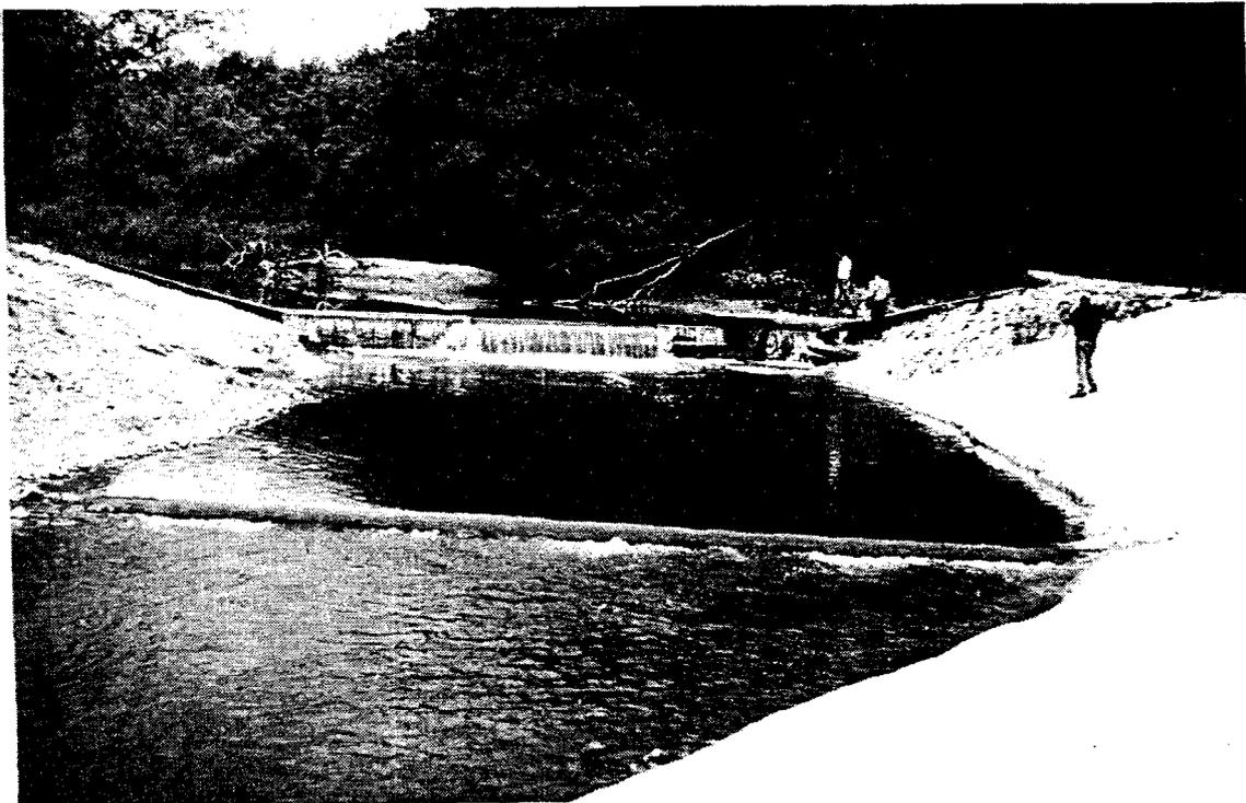
5. Sea lamprey barrier dam on Duffin Creek, Lake Ontario, Ontario. It is a low head barrier dam constructed of steel sheet piling and has a built-in lamprey trap and jumping pool. Note the structure downstream from the barrier to elevate and maintain the head of the jumping pool.
