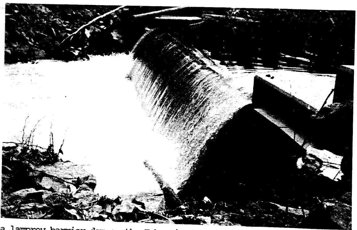
14. Sea lamprey barrier dam on the Echo River, Lake Huron, Ontario. A 1.2 m (4 ft) dam constructed in the early 1970's with timber cribs. This structure is being replaced in 1986 with a new dam constructed of steel sheet piling.
