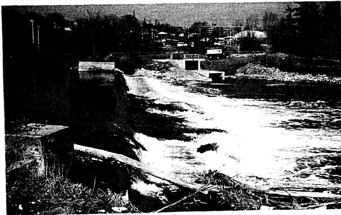
7. Sea lamprey barrier dam on the Credit River, Lake Ontario, Ontario. The barrier dam was reconstructed in 1980-81 from an existing mill dam. A fishway built by the province is shown as well.
