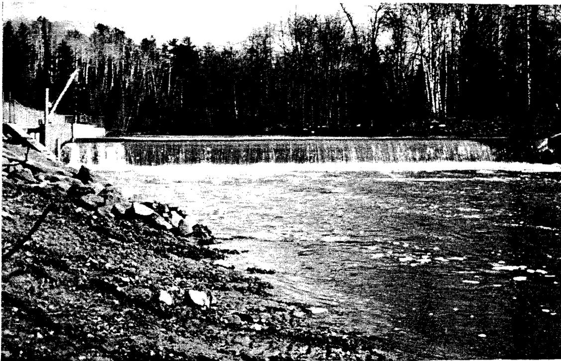
29a. Sea lamprey barrier dam on the Brule River, Lake Superior, Wisconsin. This concrete dam was reconstructed in 1986 and has a fishway with a built-in lamprey trap and observation chamber.
