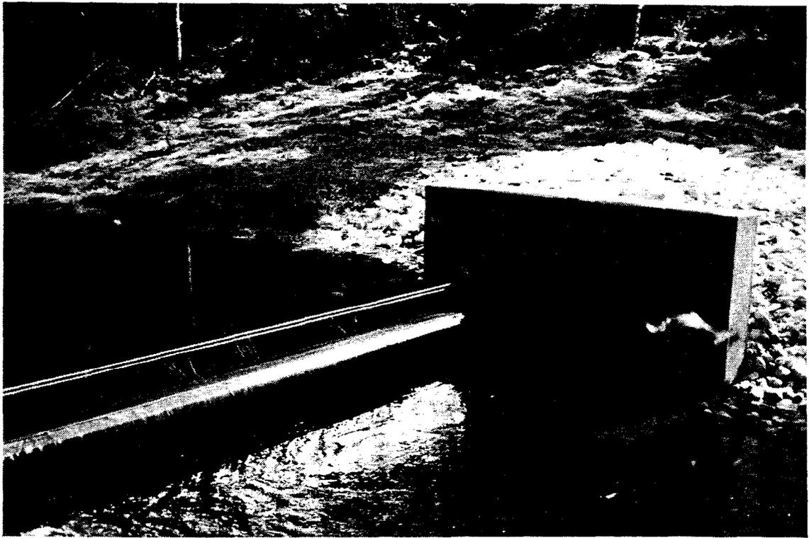
22a. Sea lamprey barrier dam on Albany Creek, Lake Huron, Michigan. The dam has a hinged gate to permit lowering during the non-lamprey migration period as well as a jumping pool and portable assessment traps. Adjustment of the height of the barrier is achieved by a cable and manual winch.
