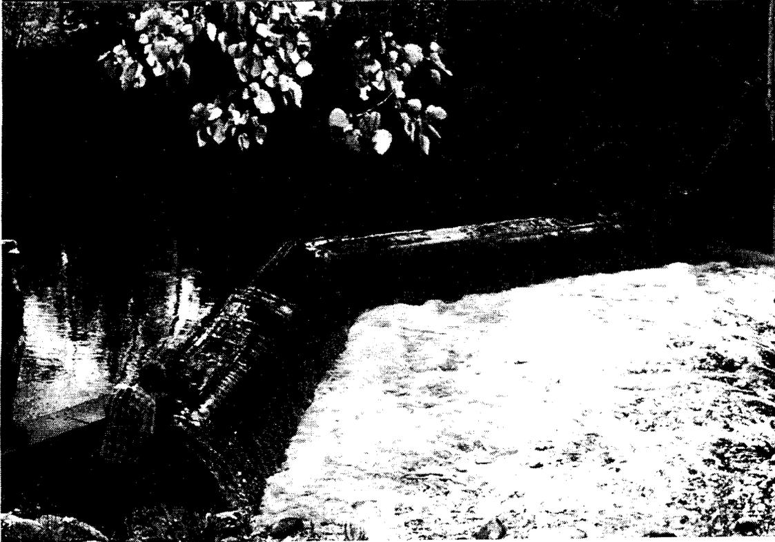
30. Sea lamprey barrier dam on the Middle River, Lake Superior, Wisconsin. It is a low head dam constructed of concrete in 1983 with a jumping pool and portable lamprey traps.
