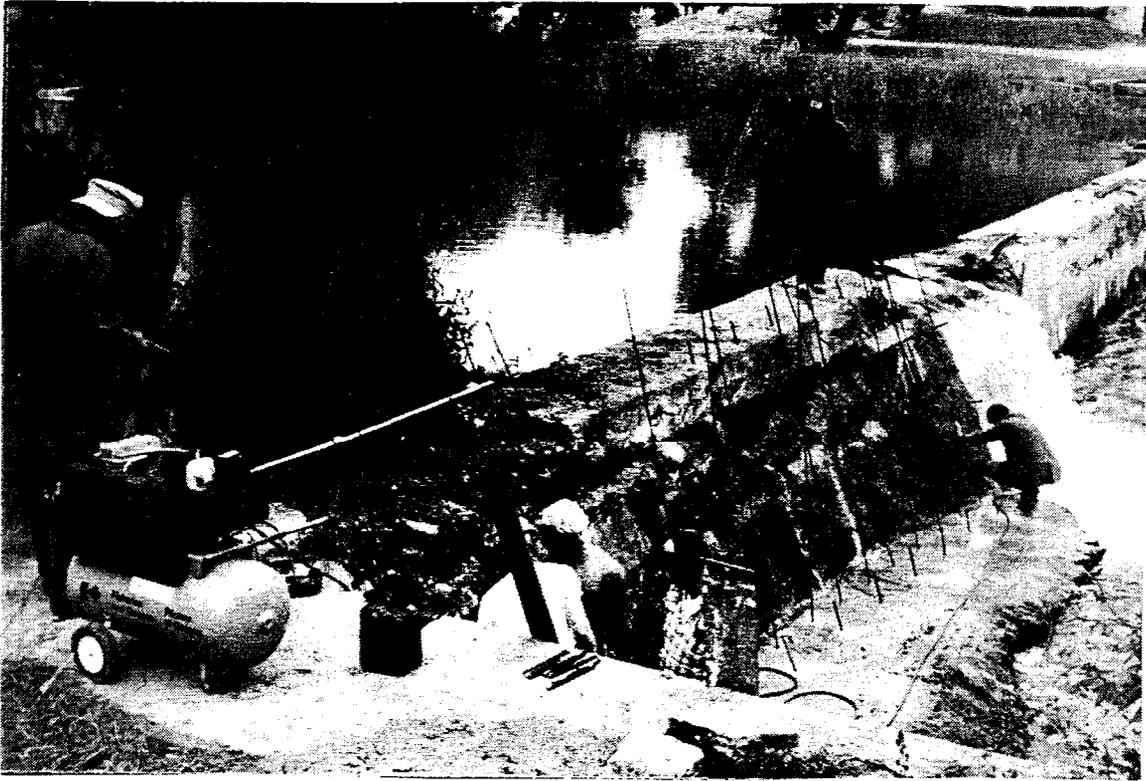
1. Sea lamprey barrier dam on the Salmon River, Lake Ontario, Ontario. Recent maintenance to the face of the old mill dam that was modified in the 1970's to block the passage of spawning-phase sea lamprey.
