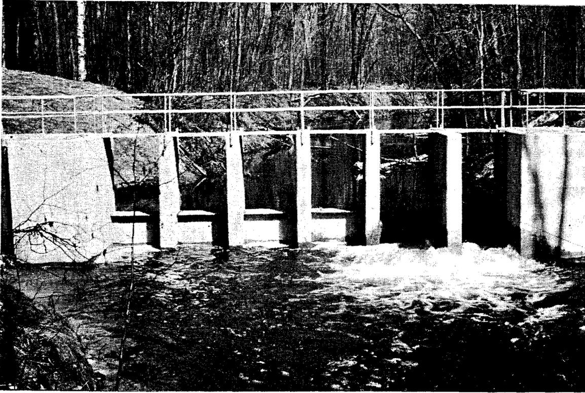
21. Sea lamprey barrier dam on the East **Branch** of AuGres River, **Lake** Huron, Michigan. A low head concrete dam constructed in 1983 with 2 stop-log bays to permit **drawdown**. In 1986 a coffer dam was constructed **downstream** to elevate the tailwater level and a jumping pool was added in the area of the stop log bays to facilitate fish passage. It has facilities for attaching portable **assessment** traps.
