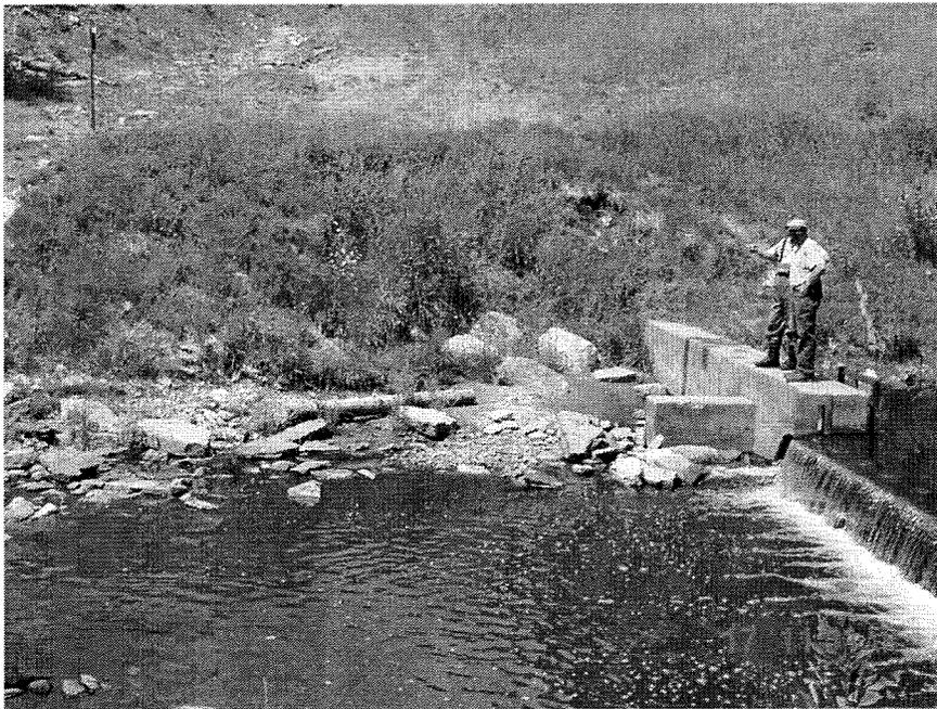
Figure 2. Different abutment and armoring designs used at sea lamprey barriers. Top. An angled, sheet metal abutment is shown on the far side of Duffin's Creek, ON. Bottom. A vertical, concrete abutment is shown on the far side of Day's River, MI.
