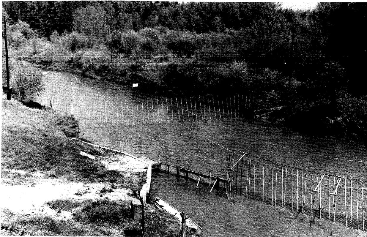
Fig. 6. Electric sea lamprey barrier and trap above the mouth of the Brule River, Wisconsin, June 1965. Water flow is from left to right. The direct-current electrodes at lower right, which extend across the river, lead fish into the trap near the stream bank (left center).
